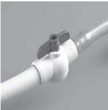
Open drain valve in equipment compartment.
