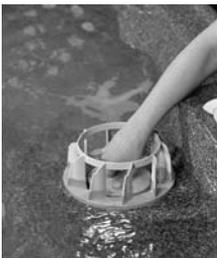
Turn filter cartridge counterclockwise to unscrew.
